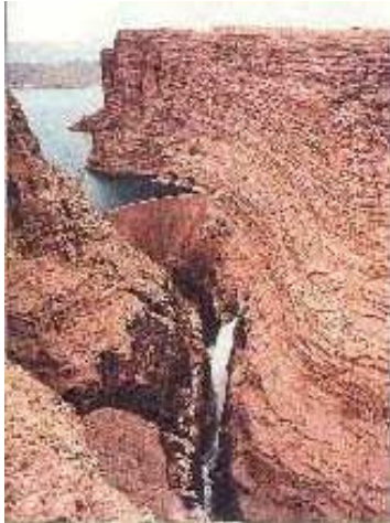
Dez Dam, Iran
