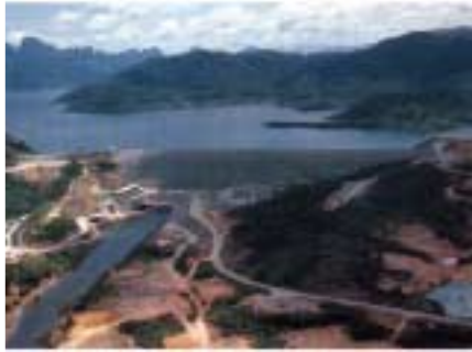
Chiew Larn Multipurpose Project, Thailand
